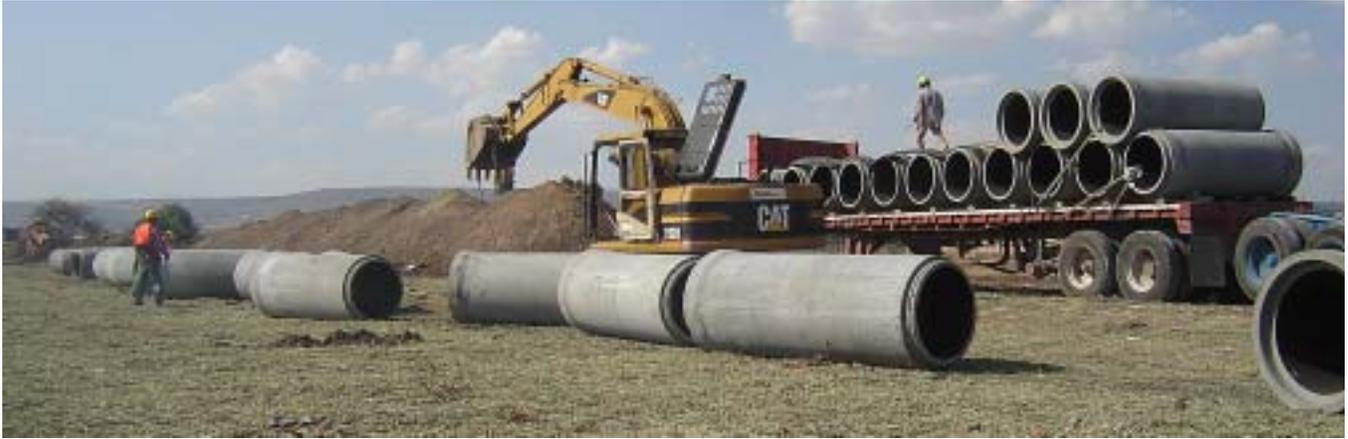
**Delivery of 30-inch and 36-inch diameter reinforced concrete pipe for three kilometer sanitary sewer.**
